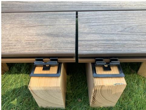
**Double joist under butt joints**
